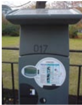
PV panels on a bus shelter roof. Solar powered parking meter.
