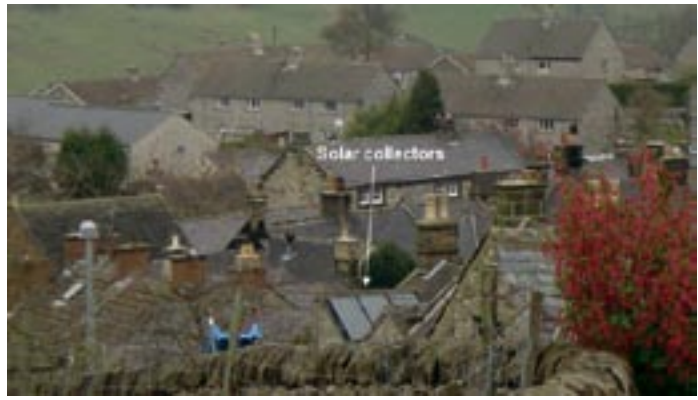
Solar thermal collectors on a house in Winster village.
